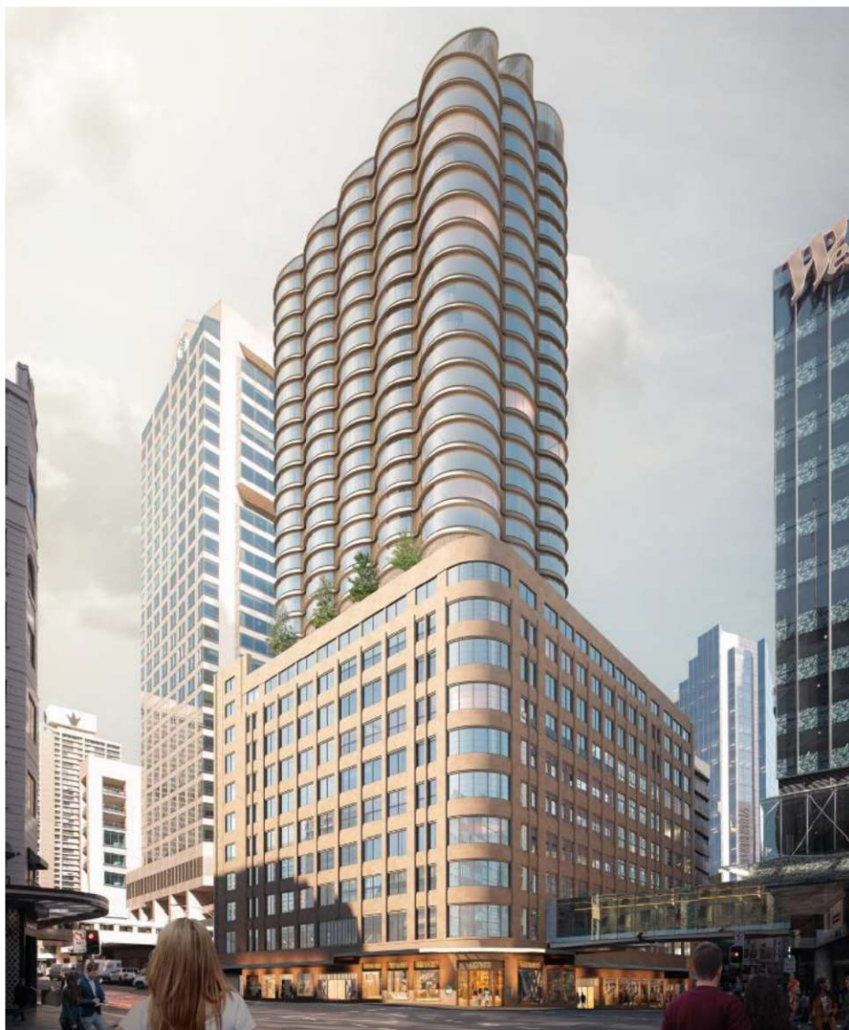
Source: Bates Smart (2018); view from NE corner of Market Street and Castlereagh Street
